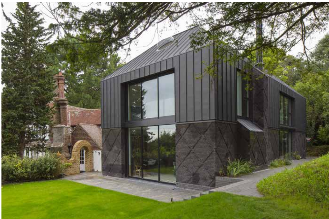
Danny Lodge (New Way Barn) West Sussex (UK) - Architecte : Matt Architecture - Technique : Joint debout VMZINC®
